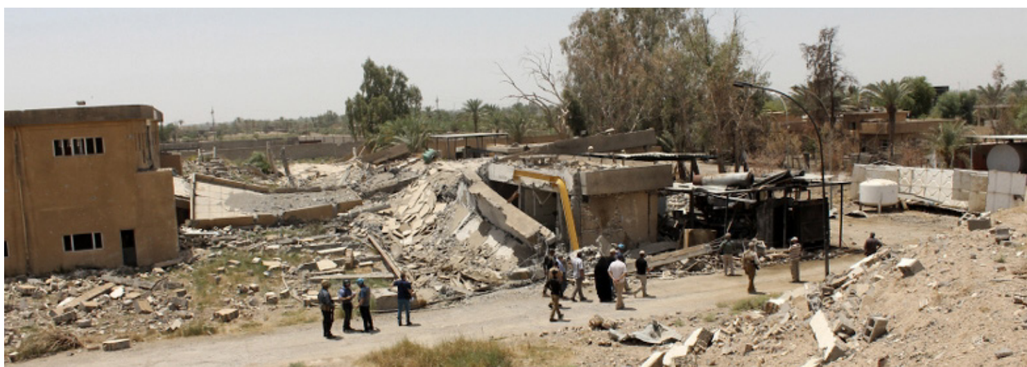
AZRAKIYA WATER TREATMENT PLANT BEFORE FFS REHABILITATION
