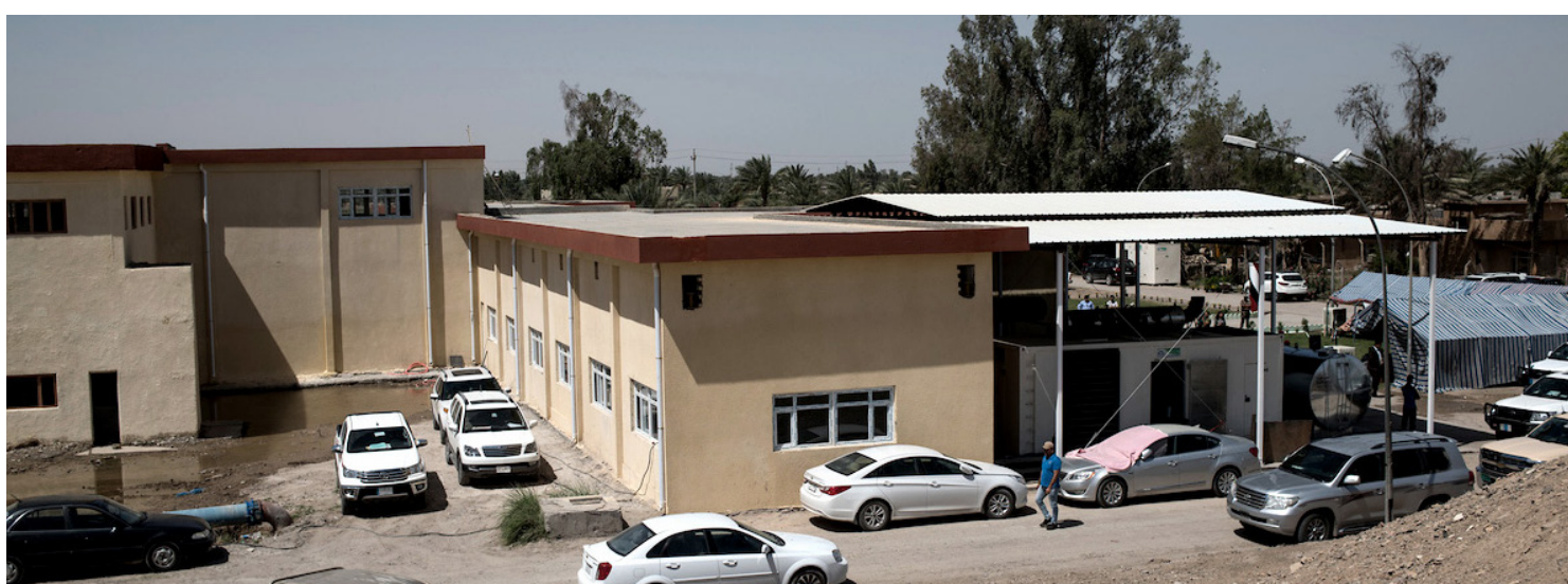
AZRAKIYA WATER TREATMENT PLANT AFTER FFS REHABILITATION
